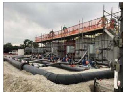
The mobile clarifier unit can handle a total suspended solids (TSS) load of up to 6,000 mg/L with integral sludge pumps that are already piped, wired, and ready for service.
